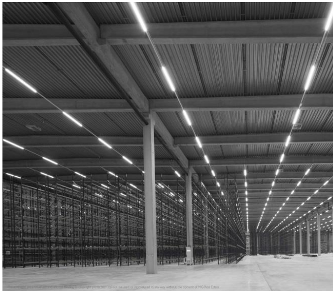
Montea «Space for Growth» - site Federal Mogul at Park De Hulst
