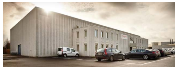
Montea "Space for Growth" - Erembodegem Site - Unit 8 (BE)
