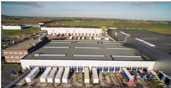
Montea “Space for Growth” – site at 's-Heerenberg (NL)
