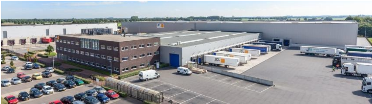
Montea "Space for Growth" – site at 's-Heerenberg (NL)
