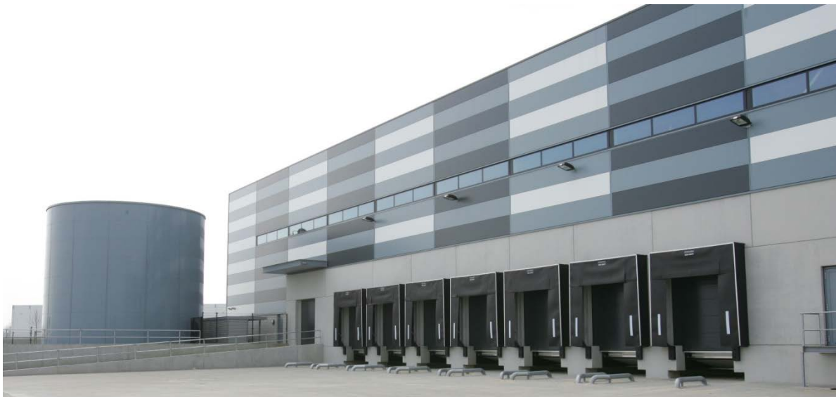
Montea "Space for Growth" – Site at Heerlen (NL)
