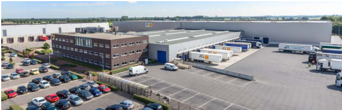
Montea “Space for Growth” – site at 's-Heerenberg (NL)
