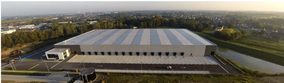
Montea «Space for Growth» - site MG Park De Hulst – Neovia Logistics Services Belgium (BE)
