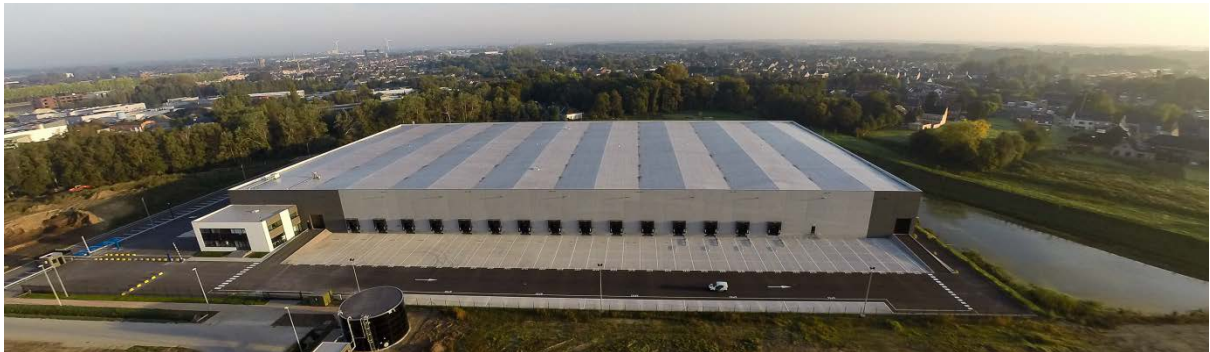
Montea «Space for Growth» - site MG Park De Hulst – Neovia Logistics Services Belgium (BE)
