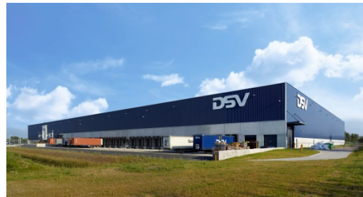
Montea "Space for Growth" – Site Haven Gent Evenstuk
