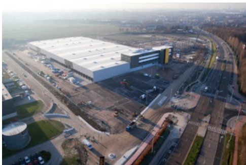
Montea «Space for Growth» - Site Brussels Airport – Brucargo West (BE)
