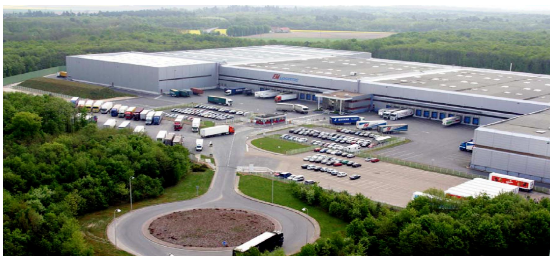
Montea « More than warehouses » - site FM Logistics - Saint-Cyr-en-Val (Orléans)
