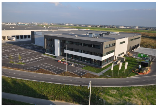
Montea "Space for Growth" – Site Brucargo 831
