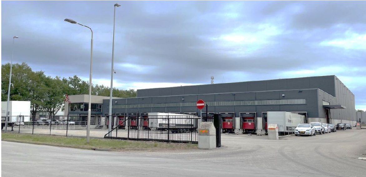
Image: ©MONTEA –Barsan Group site in Tilburg
