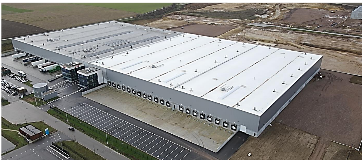
©MONTEA – Site Tailormade Logistics Tongeren – 2023
