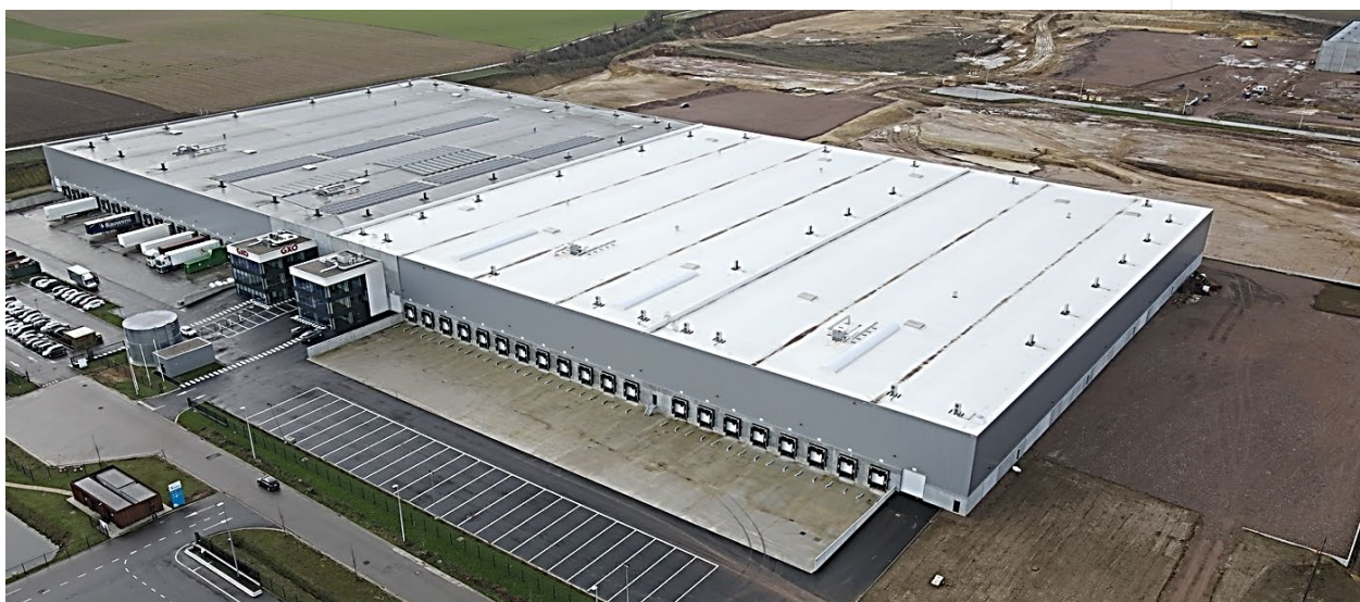
©MONTEA – Site Tailormade Logistics Tongeren – 2023
