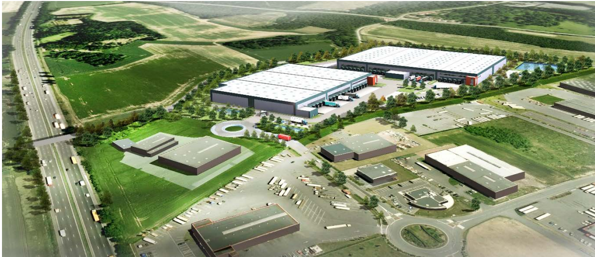
Montea "Space for Growth" - Camphin-en-Carembault site in France
