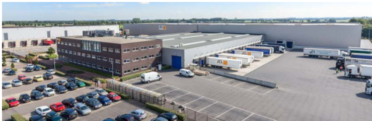
Montea “Space for Growth” – site at 's-Heerenberg (NL)
