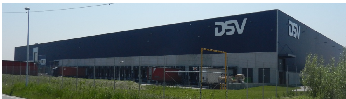
Montea "Space for Growth" – Site DSV Gent
