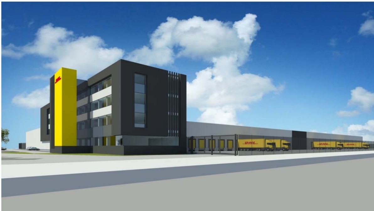
Montea “Space for Growth” – Site at Brussels Airport – Brucargo West (BE)
