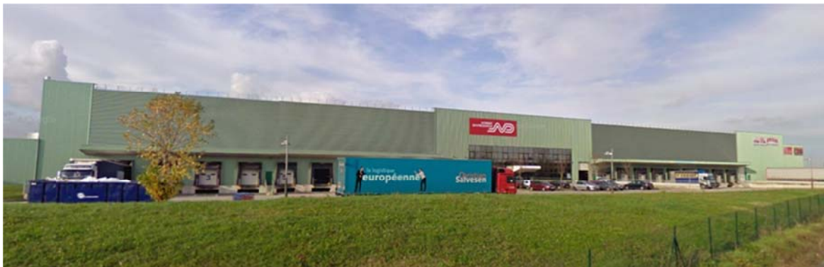
Montea « More than warehouses » - site Norbert Dentressangle | Marenes (Lyon)
