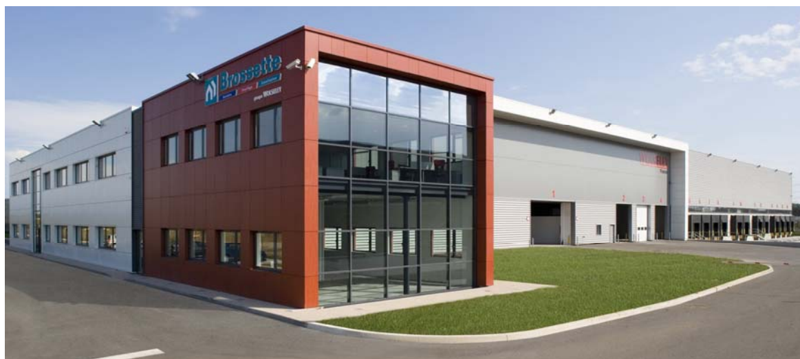
Montea « More than warehouses » - Brossette site - Saint-Priest (Lyon)
